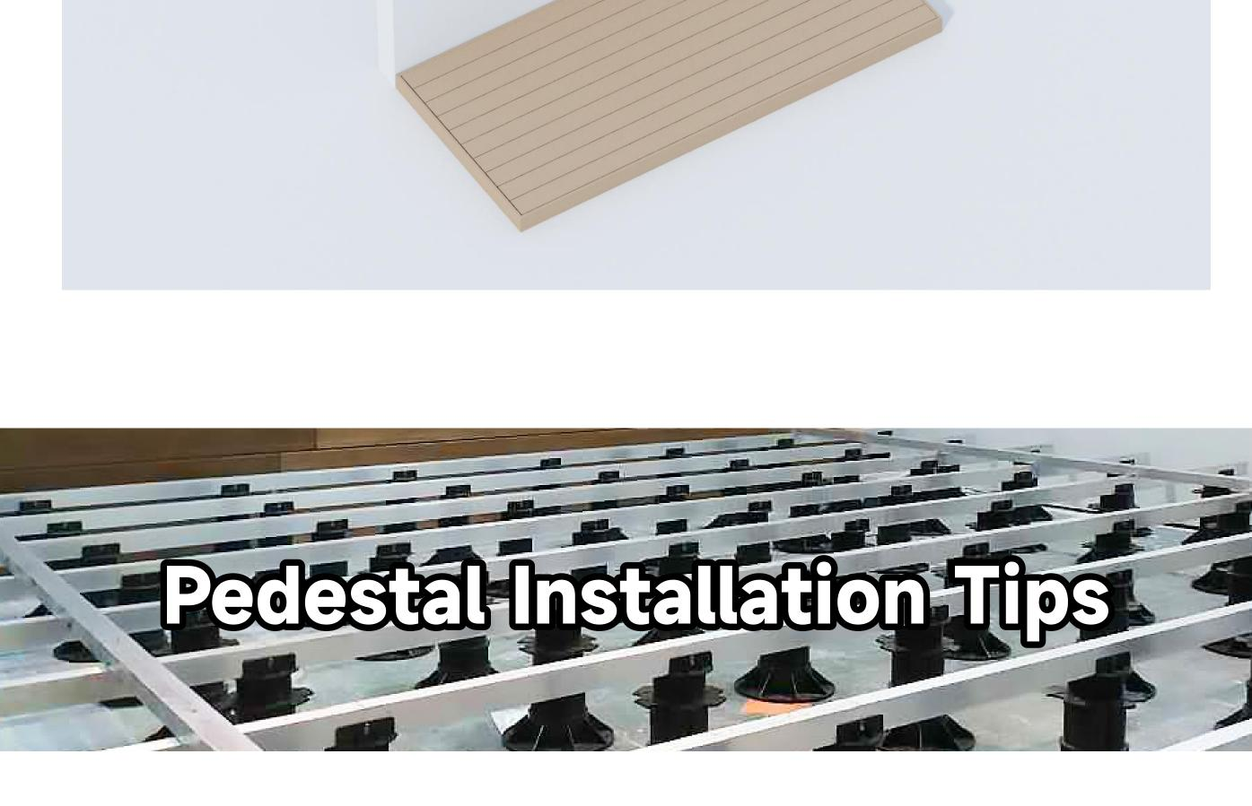
If the base of the pedestals on the edge exceeds the predetermined range, the base can be cut.
